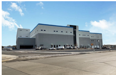
Amazon Distribution Center, Jamaica, NY
